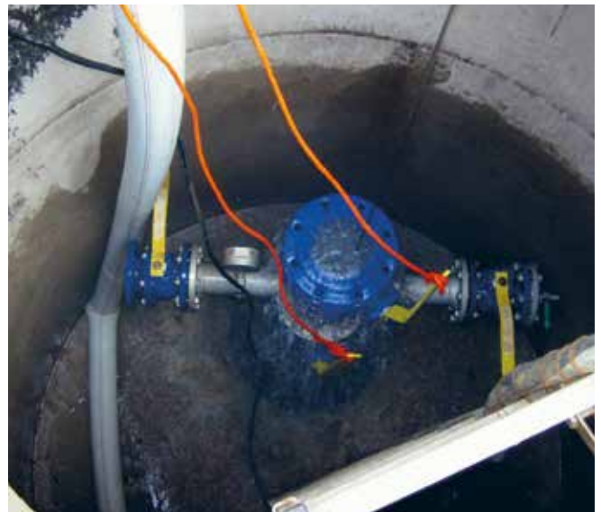
Bohrloch Engerfeld in Rheinfelden
